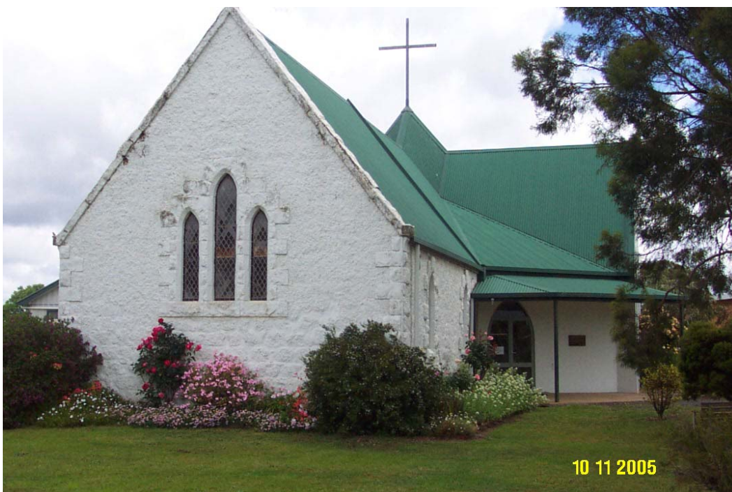
Figure 107: St. John's Anglican Church, Heywood Source: Heritage Matters Pty. Ltd.
