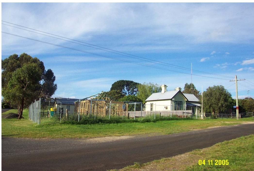
Figure 88: Dartmoor Police Station, Residence and Stables, Dartmoor Source: Heritage Matters Pty. Ltd.
