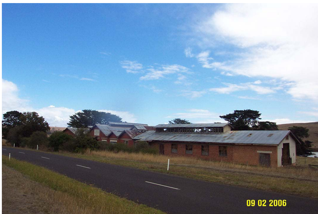
Figure 61: Merino Butter Factory, Coleraine –Merino Road, Merino Source: Heritage Matters Pty. Ltd.
