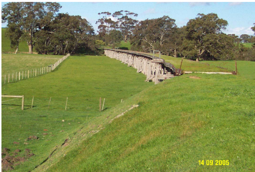
Figure 77: Casterton Rail Bridge over the Wannon, Casterton.
