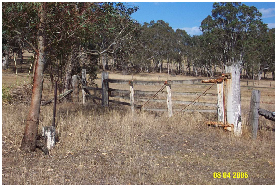
Figure 80: Railway Gates at Henty Siding, Glenelg Highway, Henty. Source: Heritage Matters Pty. Ltd.
