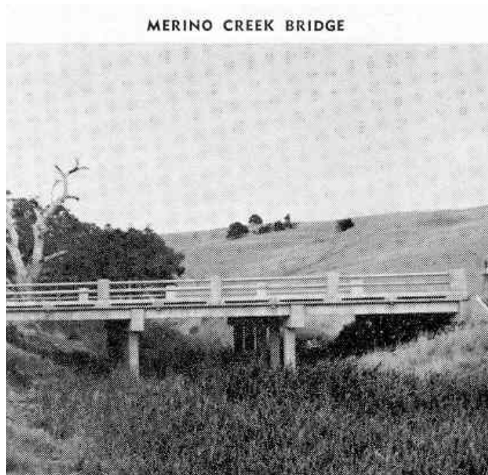
Figure 79 Merino Creek bridge, Shire of Glenelg Centenary 1963
