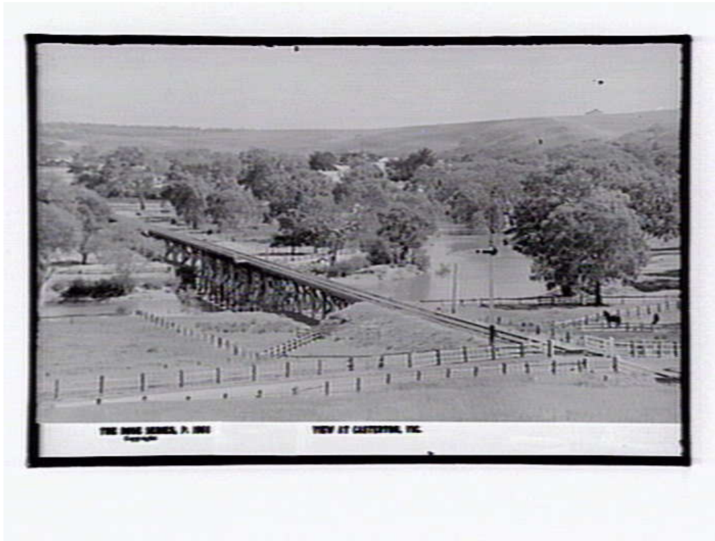
Figure 81 Casterton viaduct 1940 State Library of Victoria, Accession no H3249/2169
