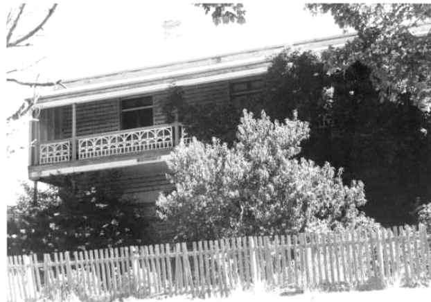
Figure 46 Nangeela State Library of Victoria Accession no H94.200/285 photo J.T. Collins
