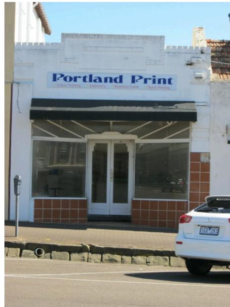
Portland Print shop (1930s), adjacent to the Star Cinema, 40 Julia Street (contributory)
