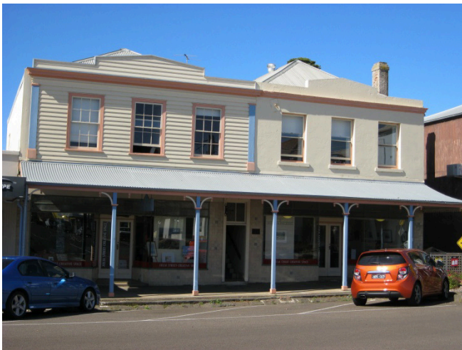
19-21 Julia Street (Shops / former Union Inn) (significant)
