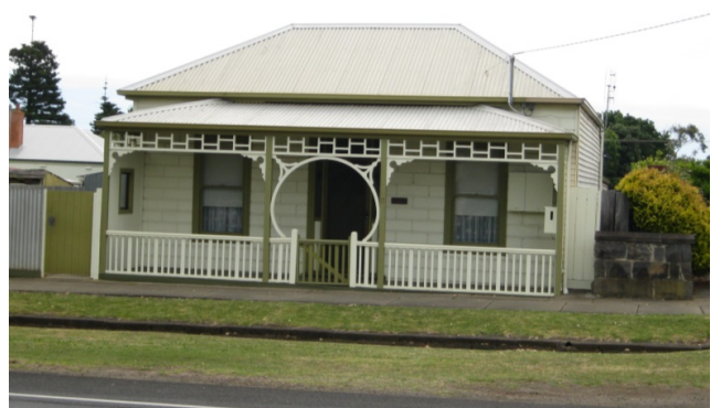
17 Hurd Street (1856, verandah detail in 1917), block fronted weatherboard with arch and timber fretwork (proposed significant)
