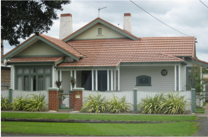
27 Hurd Street, Edwardian, large gables, rough cast chimneys, prominent bay window (contributory)
