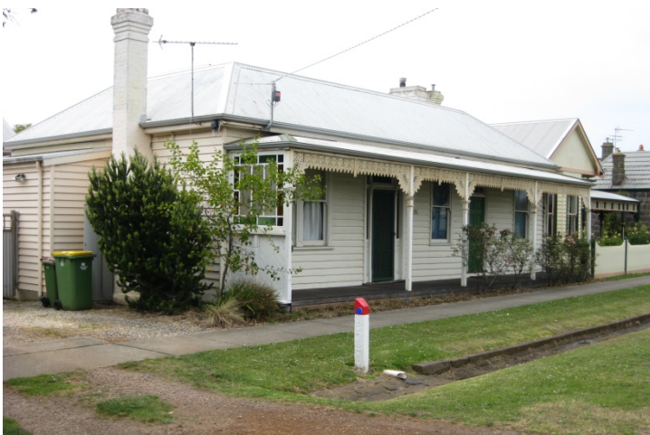
21 Hurd Street, timber cottage (1862) at front of property (significant). Note bluestone gutters in foreground
