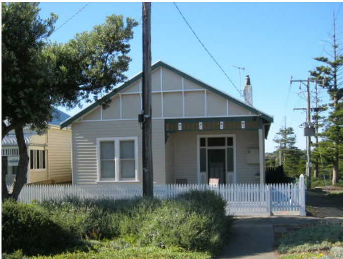
29 Gawler Street, Edwardian / Victorian weatherboard with gable roof and fine stained glass window in porch to Percy Street (contributory)
