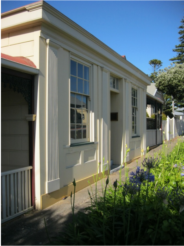
25 Gawler Street, the former Builders Arms c 1849 (significant)
