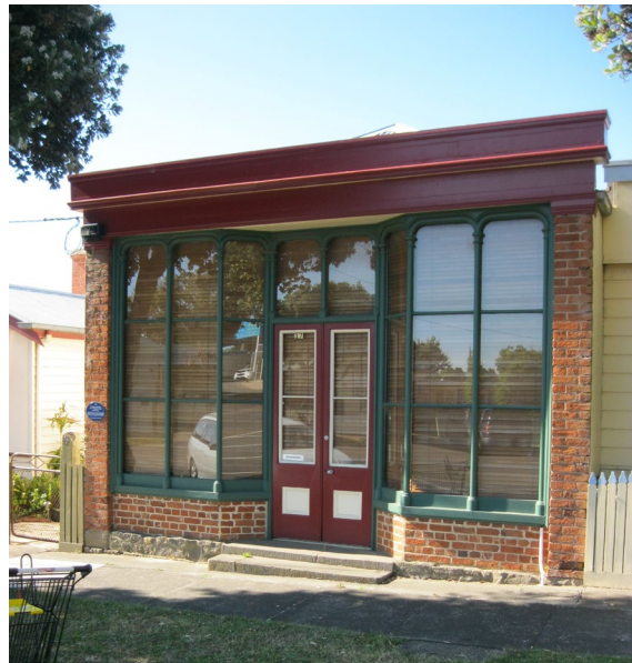
Brick and stone shop front at 17 Gawler Street, dates to around 1860 (significant)
