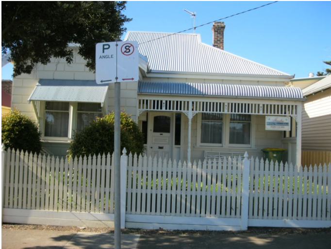
27 Gawler Street, Victorian weatherboard house with block fronted detail and Portland brick chimney at rear (contributory)
