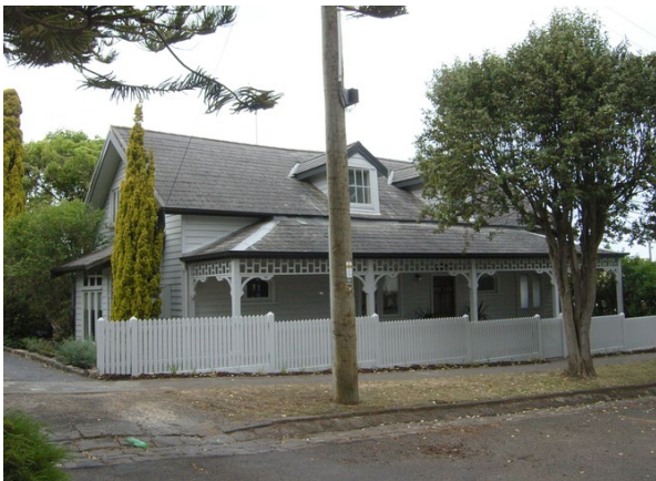
Colonial style former Portland Inn at 4 Percy Street (1840) (Victorian Heritage Database) (significant)
