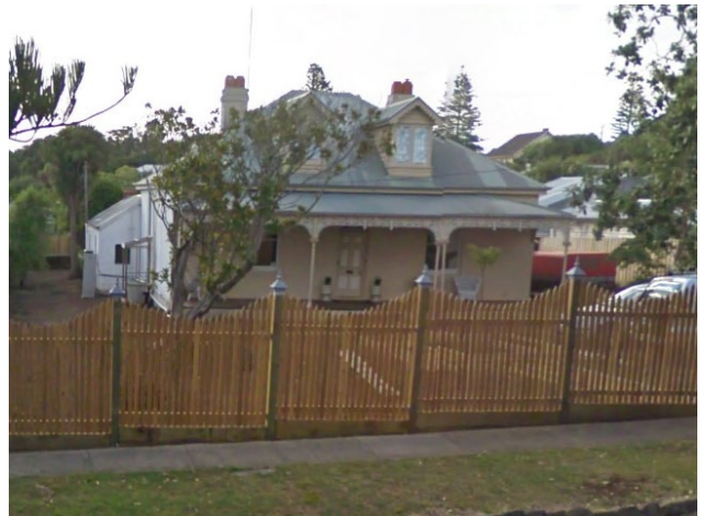
Colonial Victoria house at 5 Percy Street (pre 1857) (significant). Cast iron verandah dates to late Victorian
