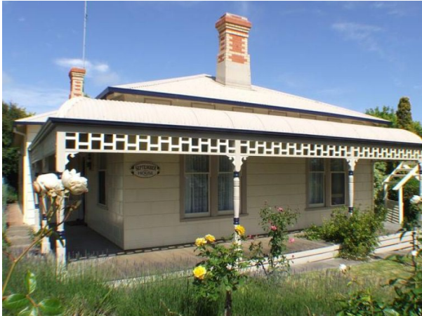
Late Victorian block-fronted weatherboard house at 6 Percy Street (1911) (significant)
