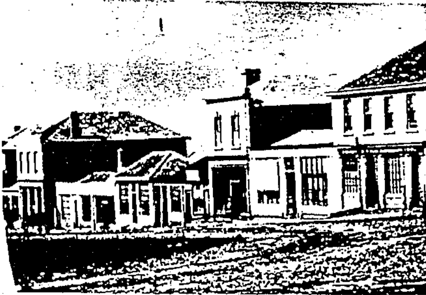
Julia Street streetscape (1850's), south side.
