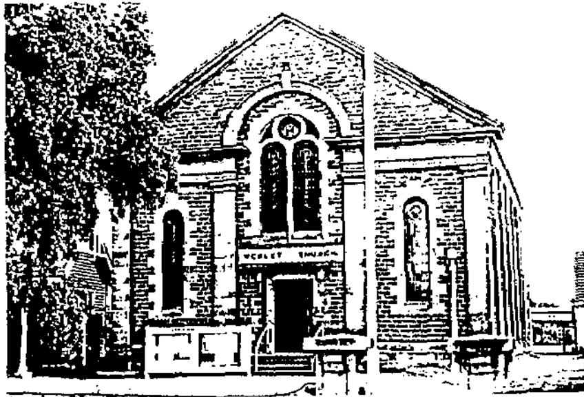
Uniting Church, former Wesleyan Church (1865), No. 61 Percy Street
