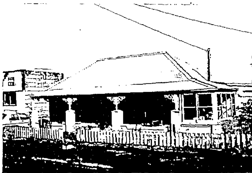
Residence, No. 30 Barkly Street.
