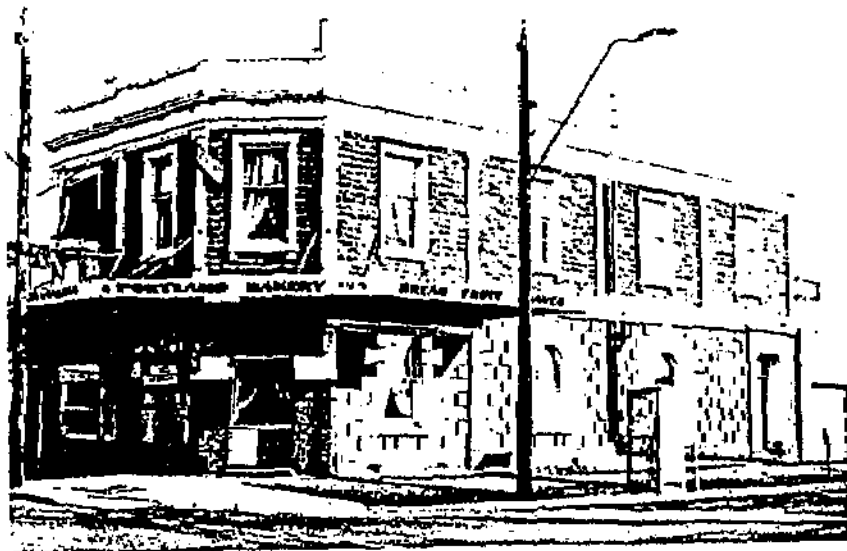
Portland Bakery, No's 79-81 Percy Street.
