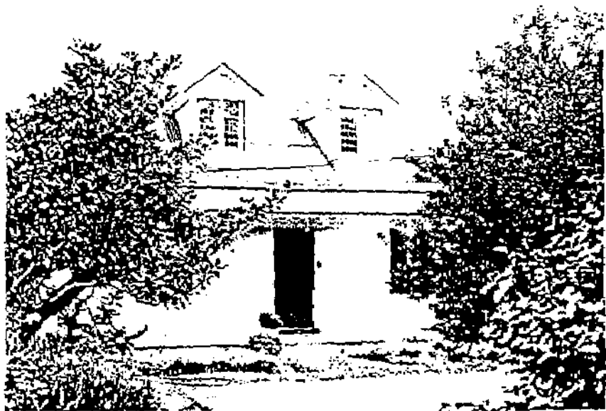
Residence, No. 5 Percy Street (pre 1857).
