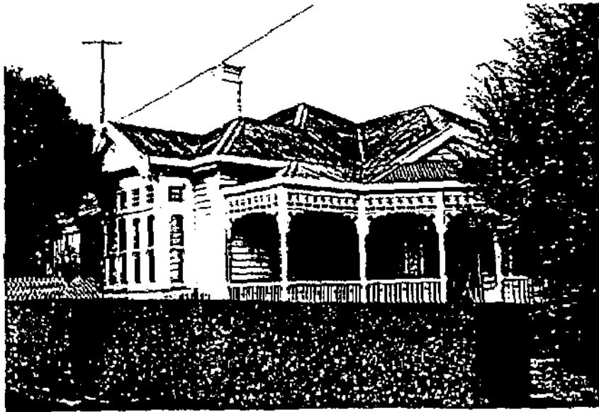
Residence, No. 138 Percy Street.
