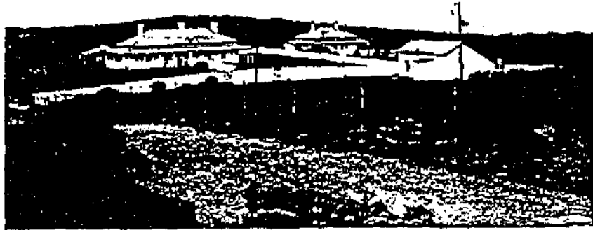
Cape Nelson Lighthouse Establishment (1883-84), Cape Nelson.
