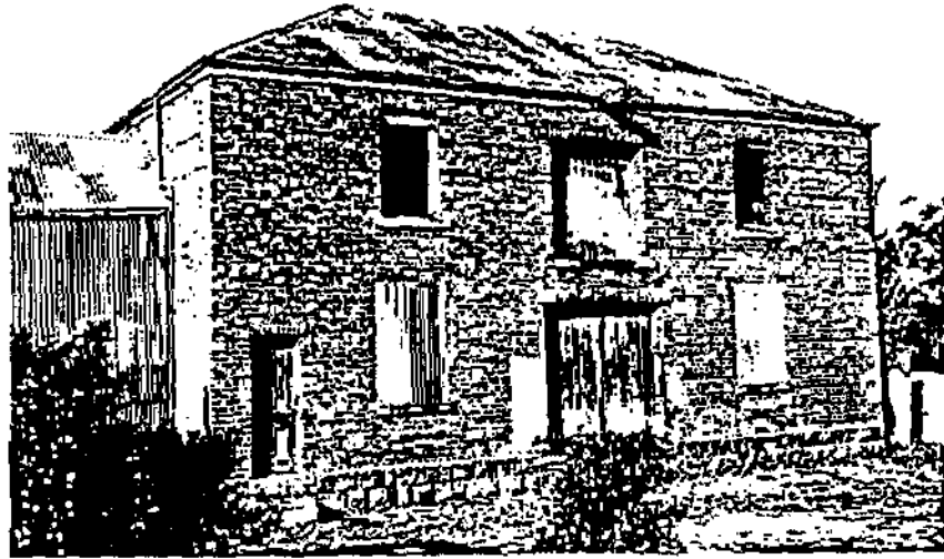
Warehouse, rear No's. 19-21 Julia Street.
