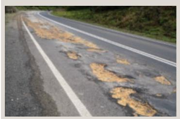
Figure 6: Failure of the road surface on Portland Nelson Road due to increasing truck volumes
