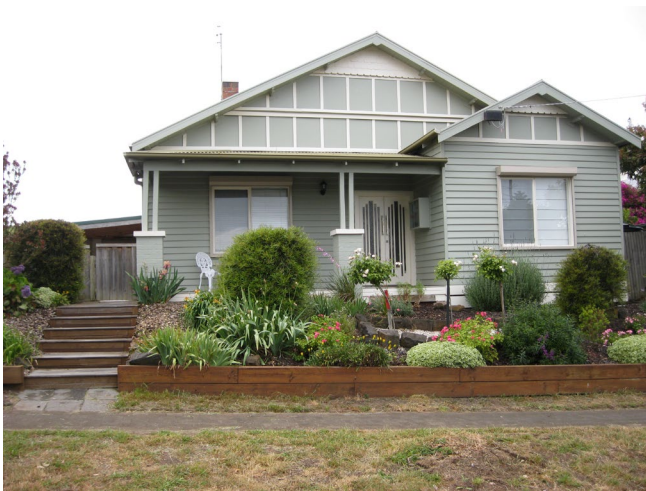
Edwardian house, 12 Percy Street
