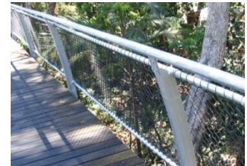
Galvanised metal handrails and black wires, mesh infill
