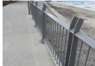
Full steel fence with rust control, powder coated finish
