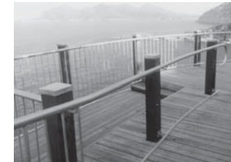
Timber posts with galvanised metal vertical post infill
