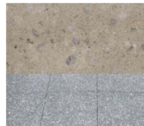
Example of cream and concrete paver combination
