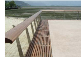
Full stainless steel fence with timber leaning rail
