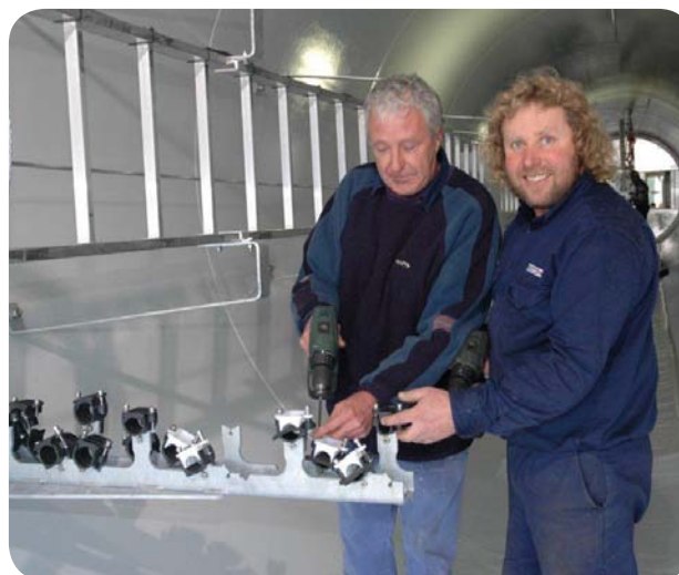
Wind tower construction
