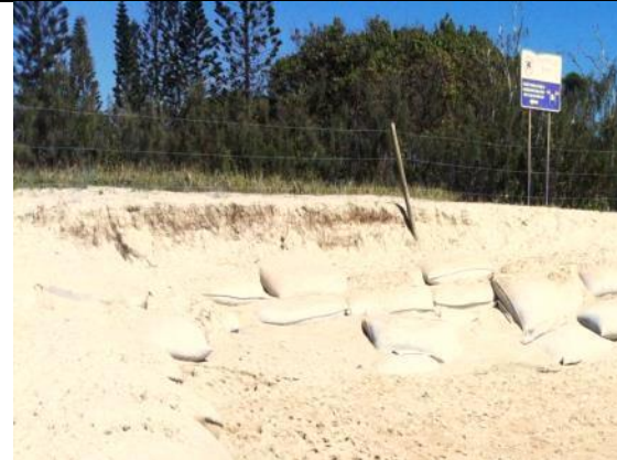
12. Sand gabions assist to protect beaches until established.
