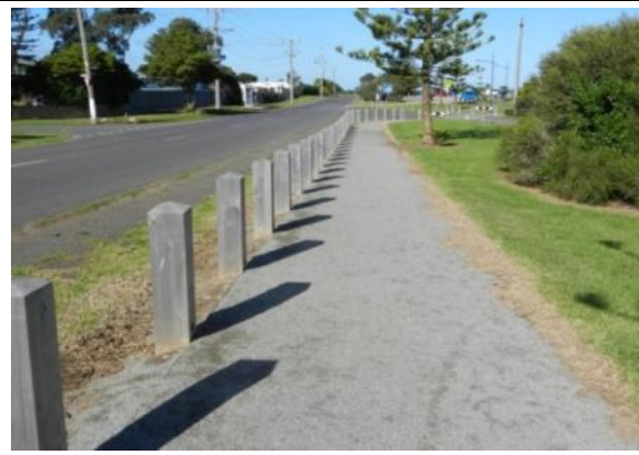
2. Bollards to separate roads from the pedestrian paths.
