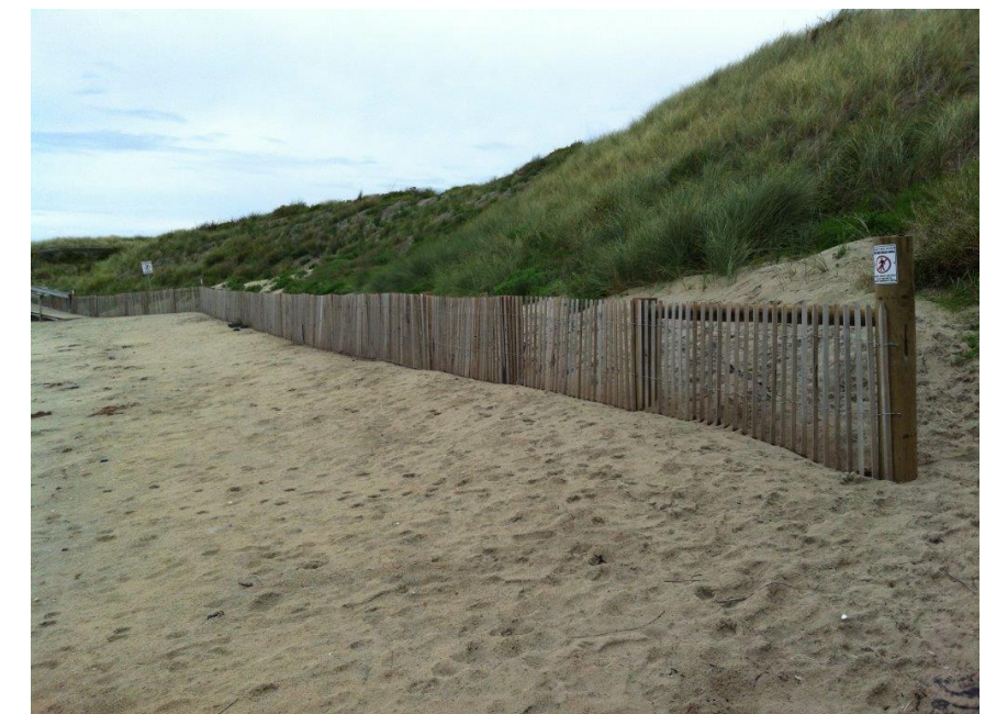
Figure 14 – Example of dune reconstruction at another coastal location.
