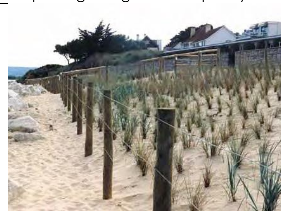
9. Resilient vegetated beaches capture natural sand drifts, protect and regenerate after storms.
