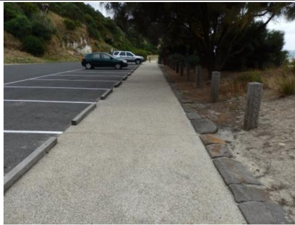
5. Car park and footpath (note timber wheel stops).
