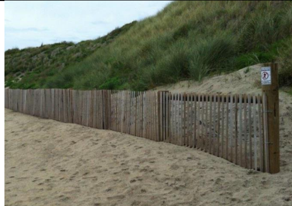
11. Beachmaster® Sand entrapment fencing assists to protect beaches.
