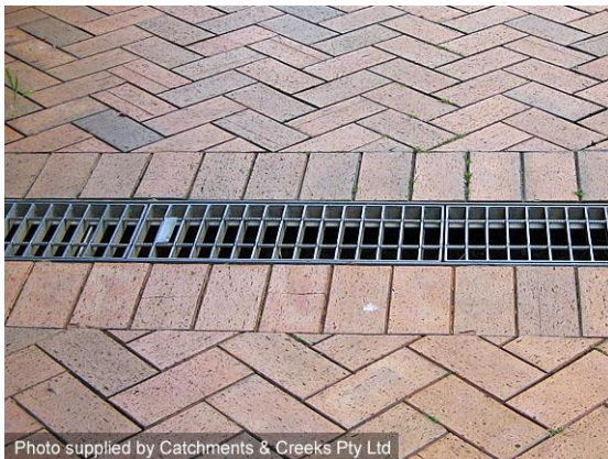
Slot drain with metal grate
