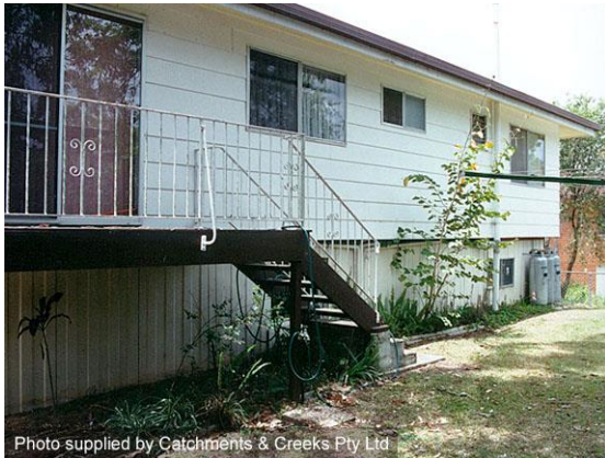
Earth fill placed against lower walls
