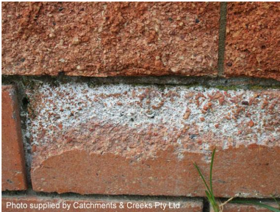
Salt damage from rising groundwater
