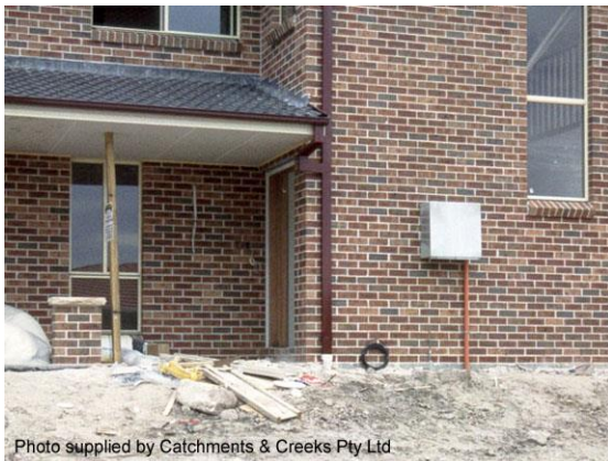
Roof water drainage on a new building
