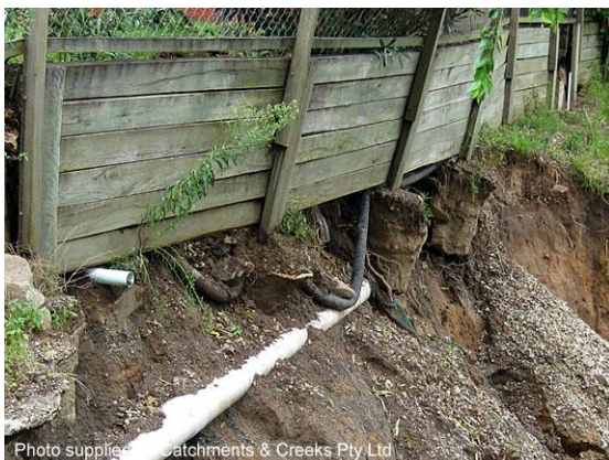
Landslip caused by stormwater discharges
