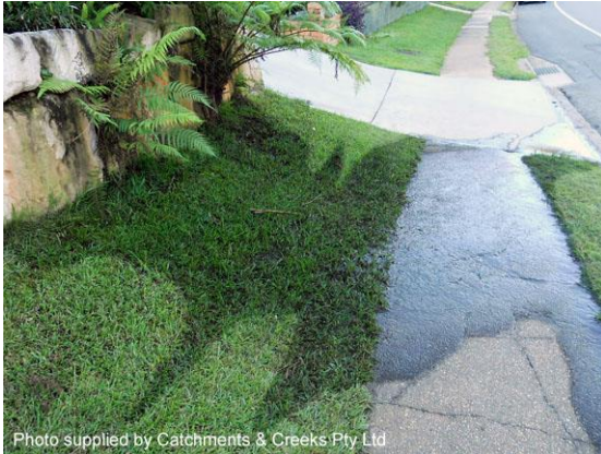
Seepage from a boulder wall
