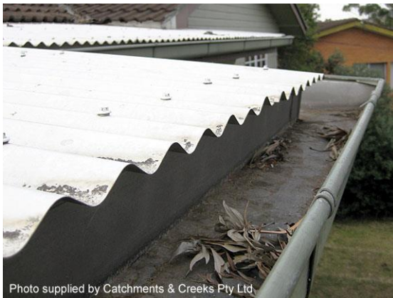
175 mm wide roof gutter
