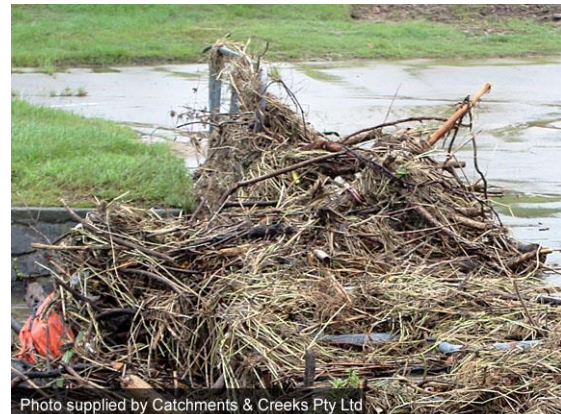
Flood debris damage to a steel fence
