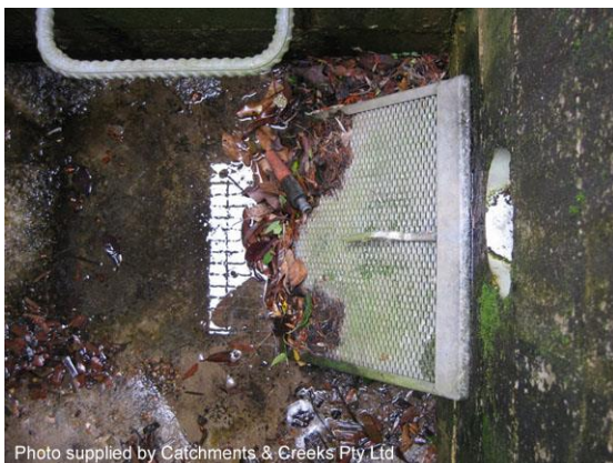
Outlet screen inside a detention tank
