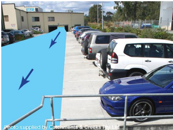
Overland flow path passing under building
