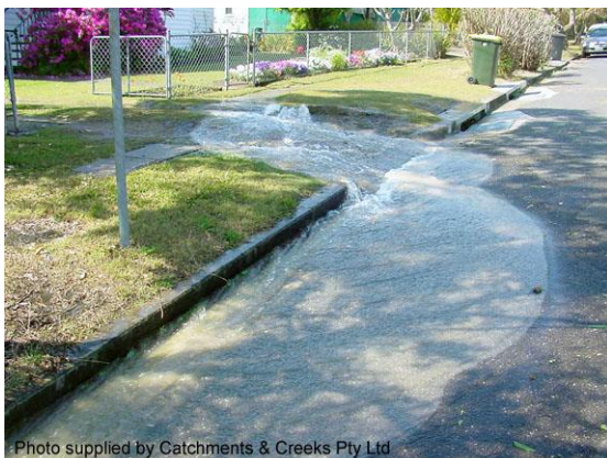
Flows caused by a water pipe failure
