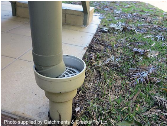
Downpipe 'connected' to the street
