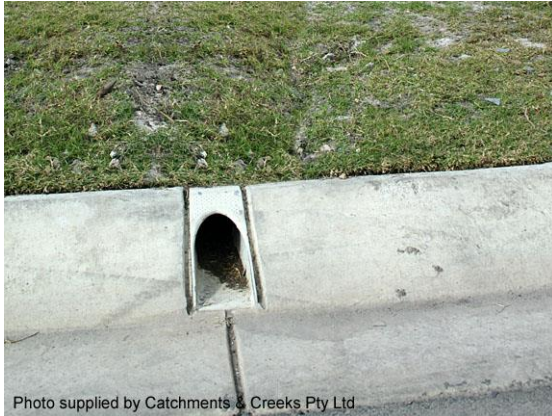
Drainage outlet to a street
