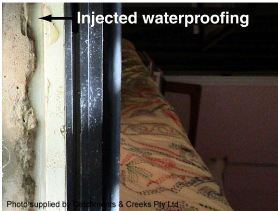
Injection of waterproofing sealer
