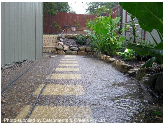
Recessed pathway carrying overland flow
