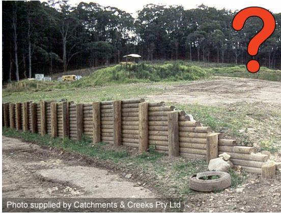
Treated timber post wall
