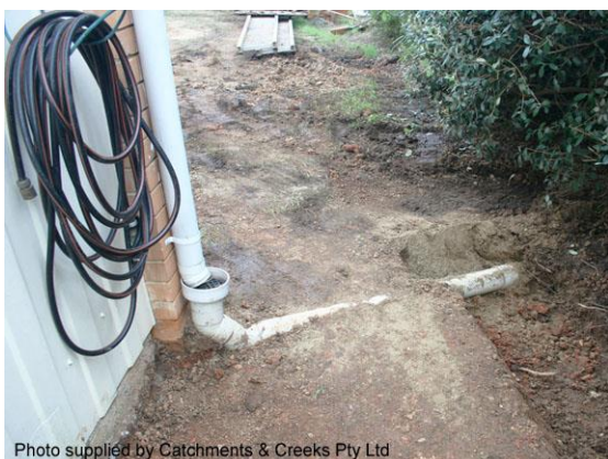
Installation of roof water drainage system
