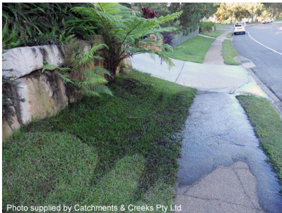
Groundwater seepage from a retaining wall
