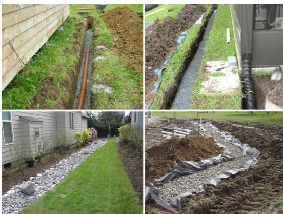
Soakage drains under construction
