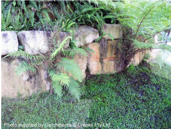
Groundwater seepage from a stone wall
