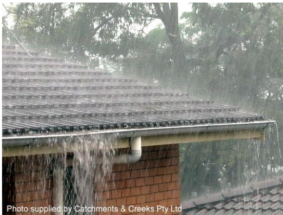
Overflowing roof gutter
