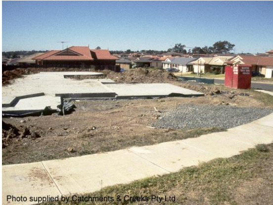
The base slab of a new home
