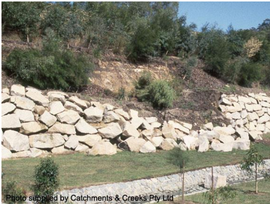
Failed rock retaining wall (landslip)
