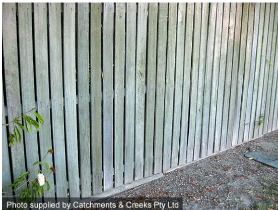
Timber fence with well-spaced palings
