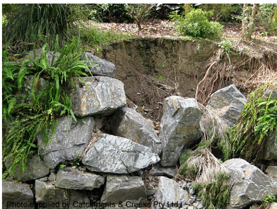
Failure of rock retaining wall
