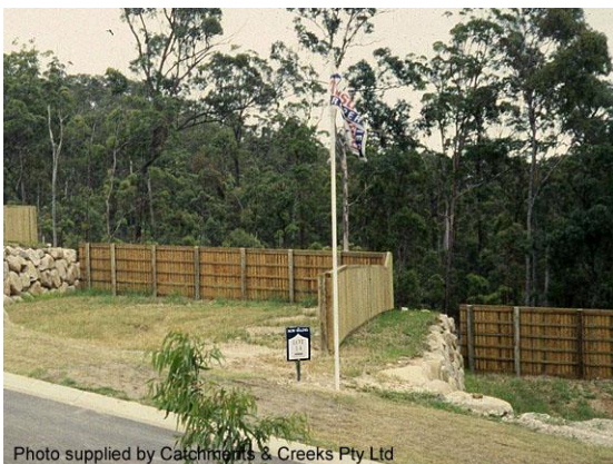
Inter-allotment retaining walls
