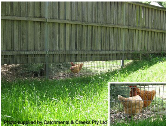
Raised fencing with lower wire mesh
