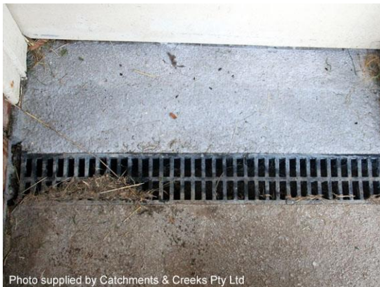
Slot drain placed in front of doorway
