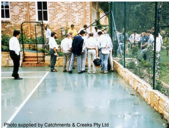
Stormwater detention using a tennis court
