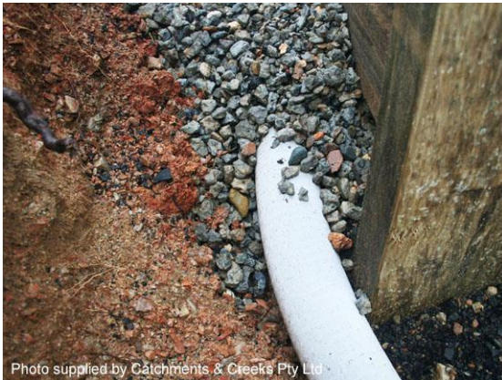
Subsoil drainage behind a retaining wall
