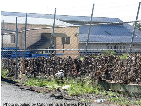
Flood debris blockage of mesh fence
