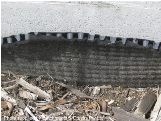
Drainage 'blanket' placed against a wall
