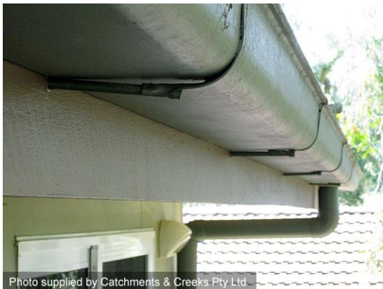
External, saddle-type bracket
